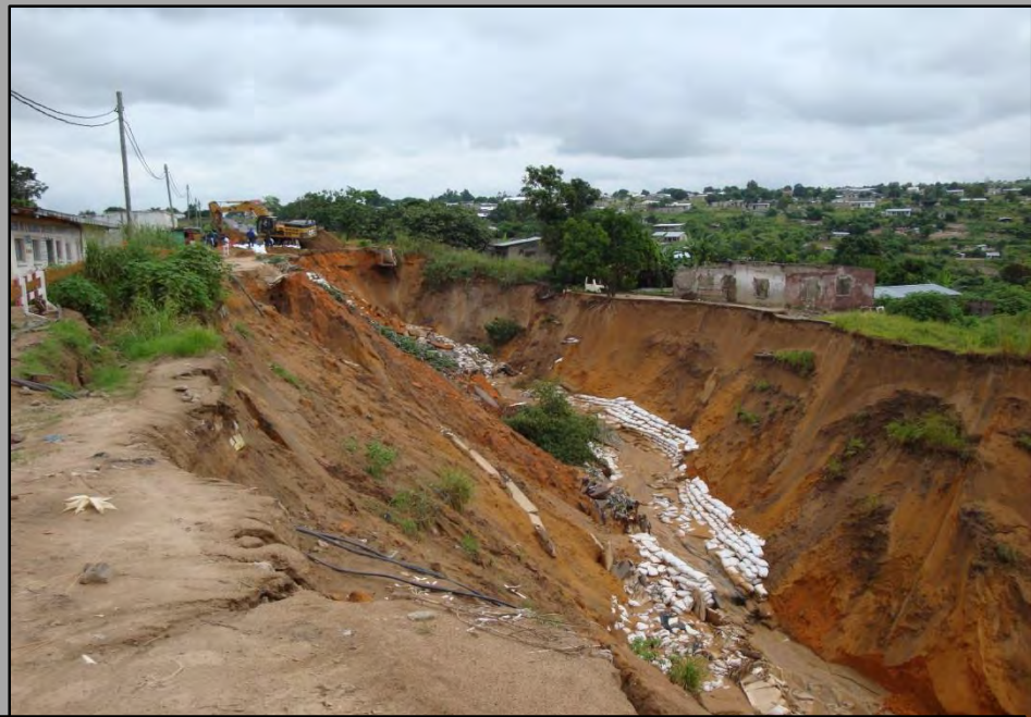
Collapsed infrastructures on Roads & Drainage channels resulting in formation of extensive gullies
