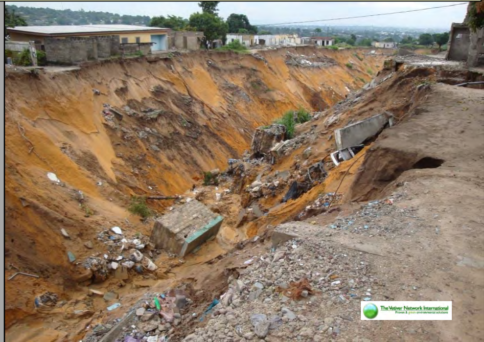
Collapsed infrastructures on Roads & Drainage channels resulting in formation of extensive gullies
