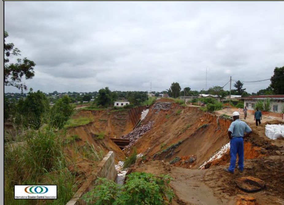
Collapsed infrastructures on Roads & Drainage channels resulting in formation of extensive gullies
