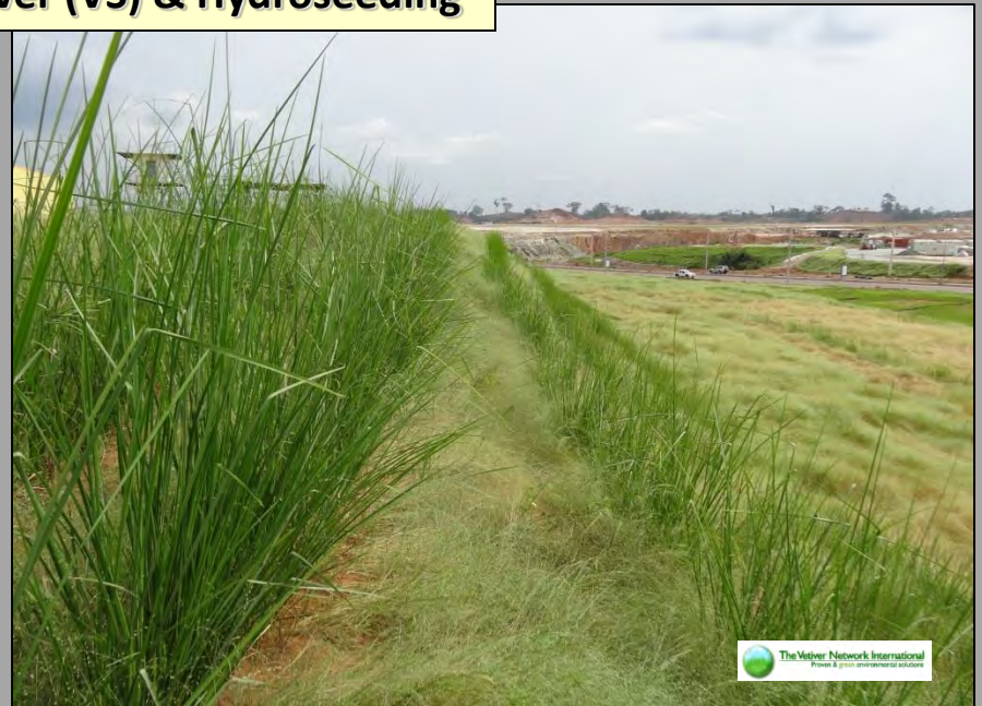
Established Side Slopes using Vetiver (VS) & Hydroseeding
