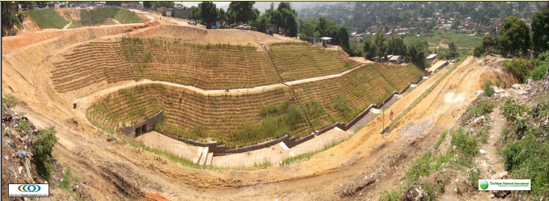
Construction activities and finishing off of side slopes in progress on newly constructed drainage system
