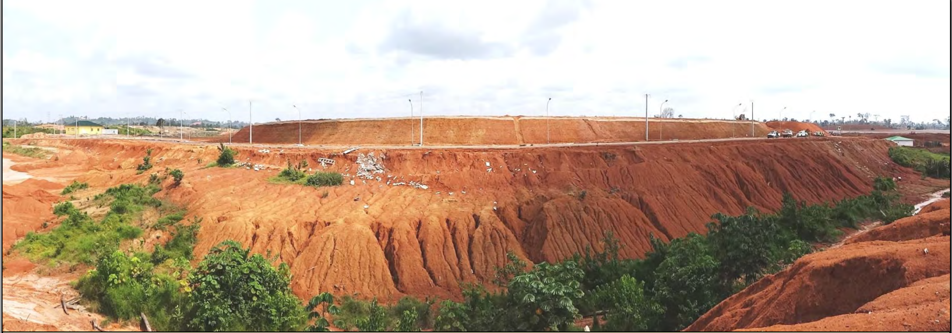
Before & After pictures of the VS for slope stabilisation – Reasonable cover attained on lower slope
