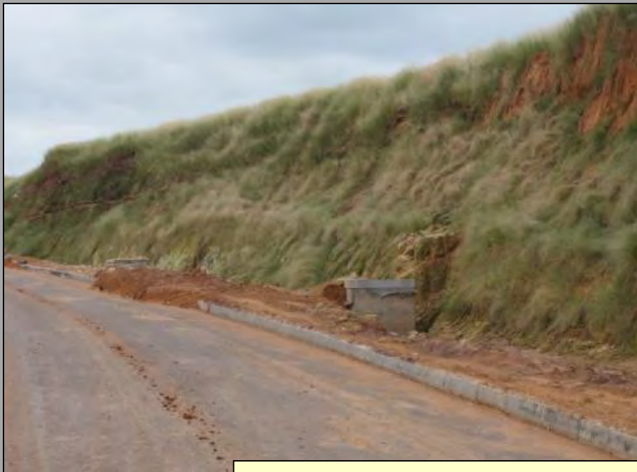
Established Side Slopes using Vetiver (VS) & Hydroseeding
