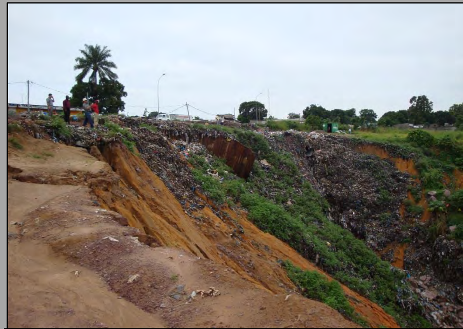
Collapsed infrastructures on Roads & Drainage channels resulting in formation of extensive gullies
