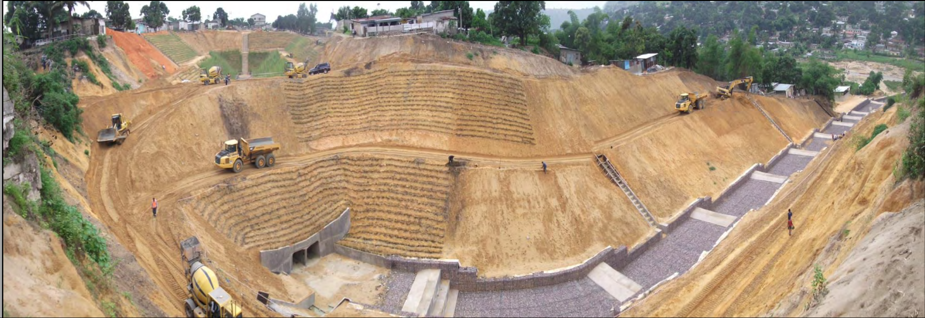
Construction activities and finishing off of side slopes in progress on newly constructed drainage system
