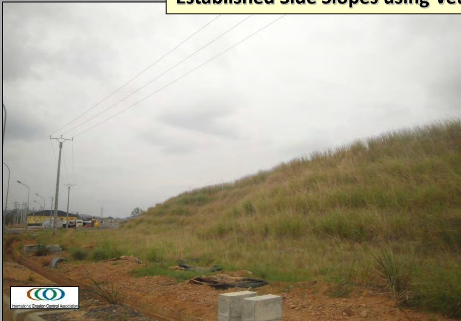
Established Side Slopes using Vetiver (VS) & Hydroseeding
