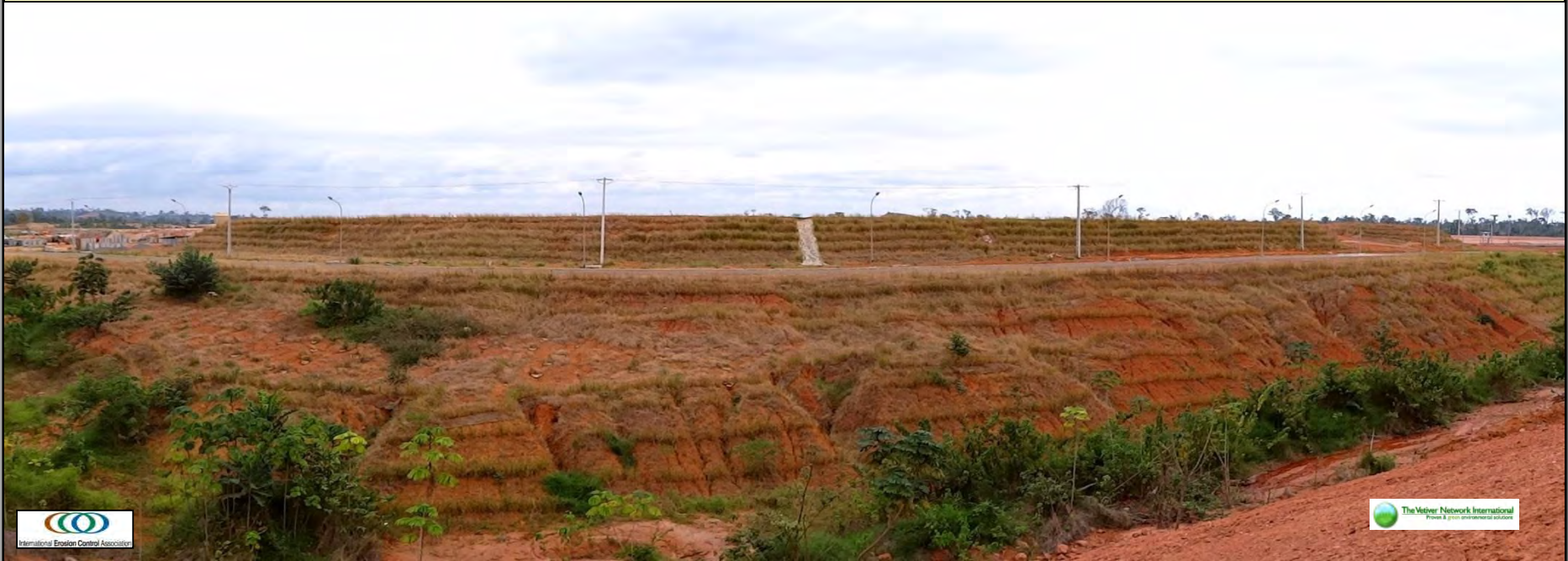
Before & After pictures of the VS for slope stabilisation – Reasonable cover attained on lower slope
